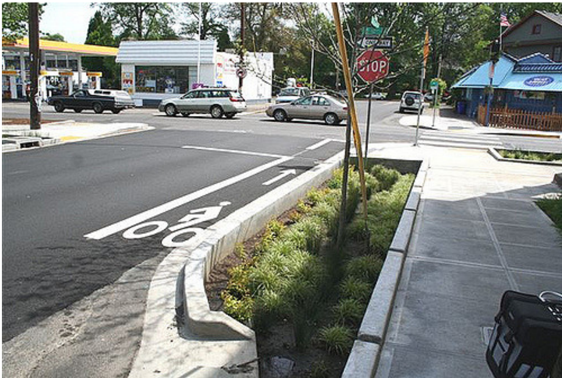
Figure 4: A small bioswale in an urban area. The pavement dips slightly down towards the curb, causing water to flow into the planted area, where it slowly filters back into the ground. (Image from Greg Raisman, Flickr).
