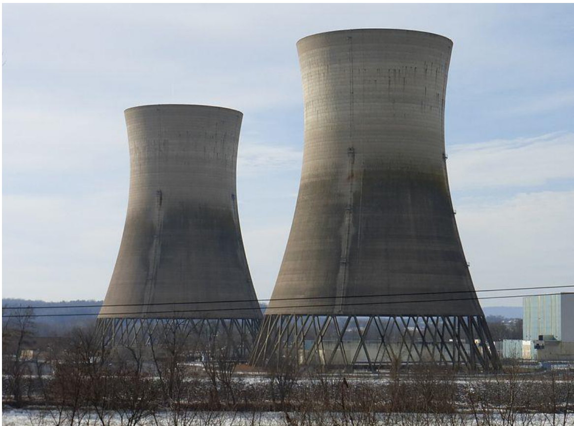
Figure 2 - Cooling Towers of Three Mile Island. The iconic, vase-shaped structures associated with nuclear reactors are actually not for generating power, but for cooling wastewater. (Photo: Wikimedia Commons).
